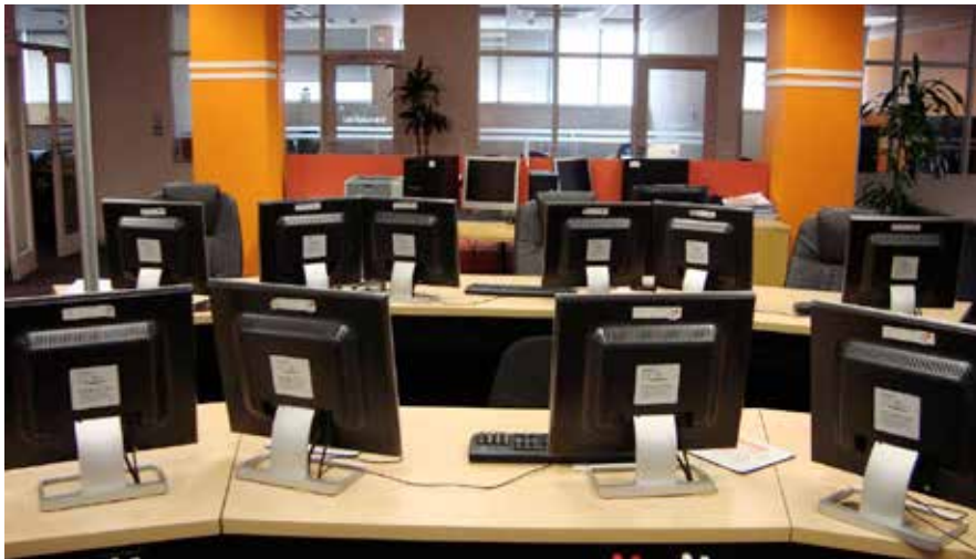
Computer equipment supplied by the consultant remains unused at the IFM and ITS systems' control room (view from the front)
